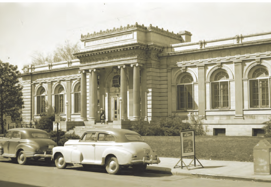
Little Rock Public Library funded by Carnegie Foundation in 1910
