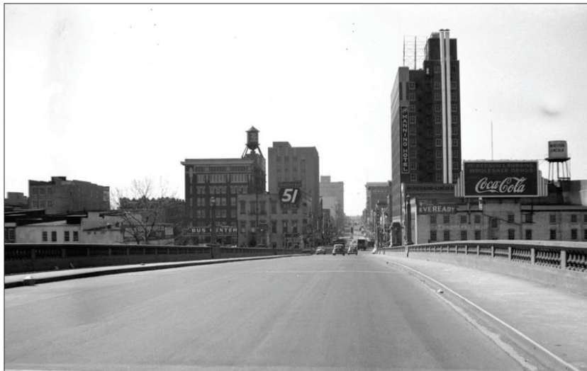
Looking south down Main Street Bridge into Little Rock, Ark., 1950.
